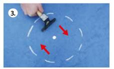
Use a hammer to spread the Linoleum Doctor fluid by gently knocking on the floor covering in one direction. Afterwards repeat in the opposite direction.
