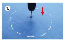
Drill a hole of 4 mm diameter in the middle of the bubble.
