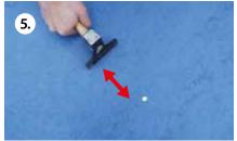
Rub the floor covering down on the whole bubble forcefully with a hammer.
