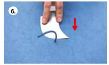
Warm a piece of linoleum welding rod in the matching colour. Put it into the drill hole then cut the excessive welding rod.
