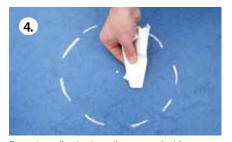
Excessive adhesive is easily removed with an absorbent cloth. Eurocol Linoleum Doctor is solvent-free, water-soluble, gentle to the skin and absolutely harmless to the floor covering.
